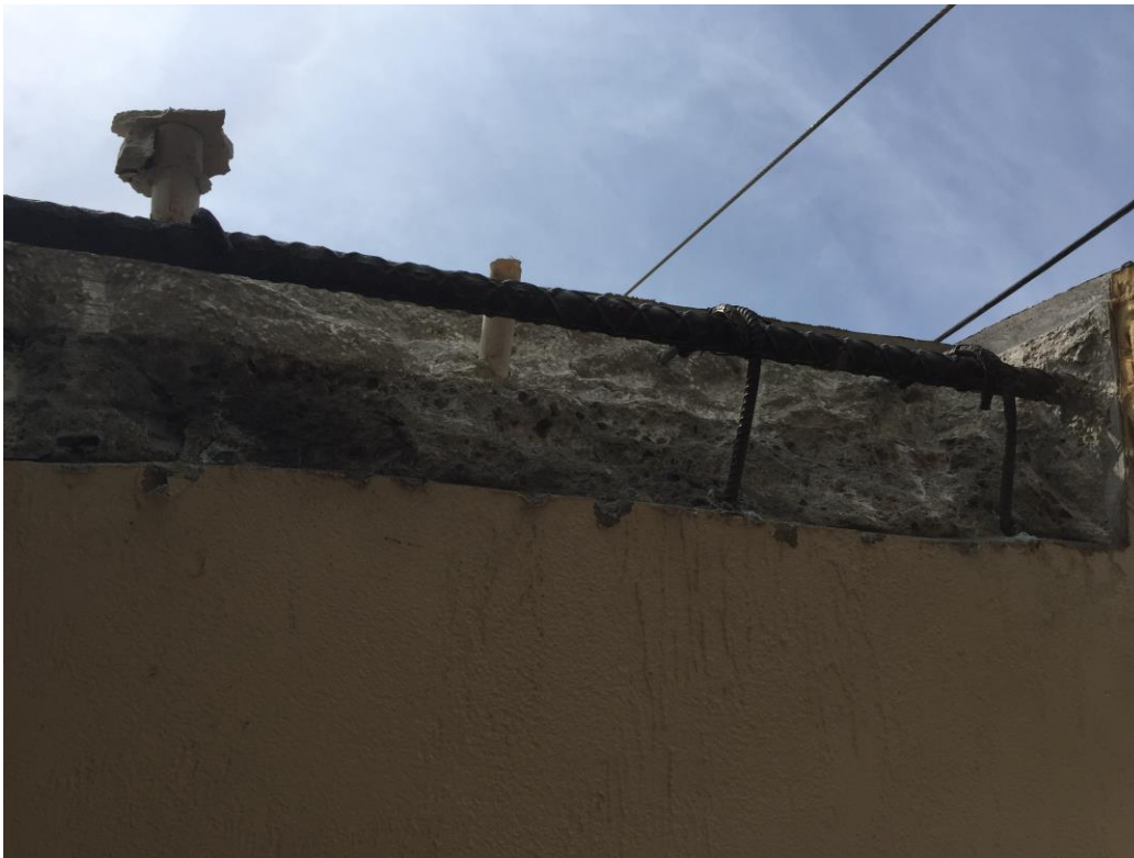
Picture 2: Typical ceiling excavation
