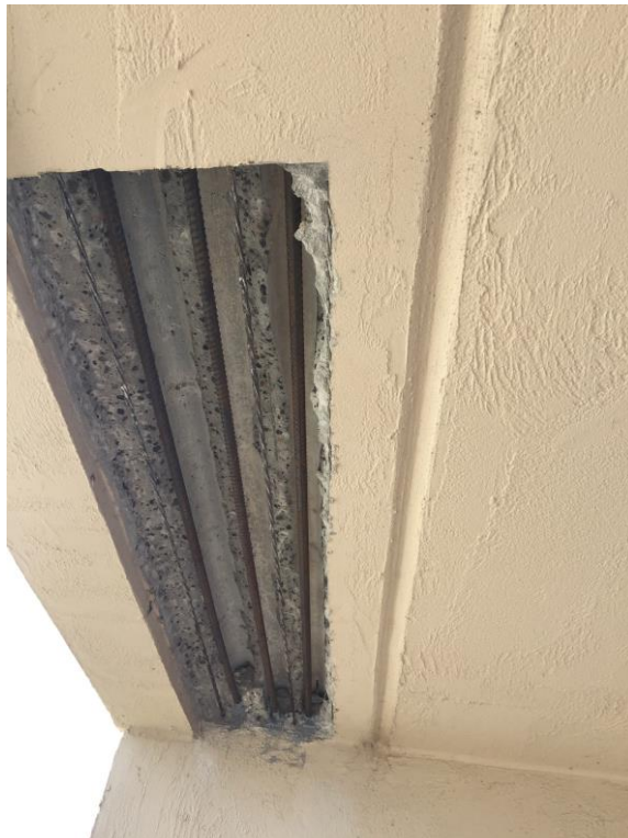
Picture 4: Typical ceiling excavation
