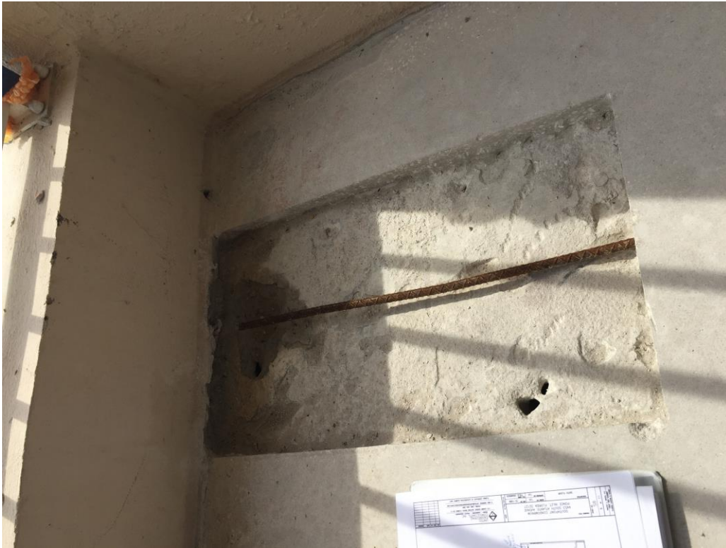
Picture 1: Typical topside excavation
