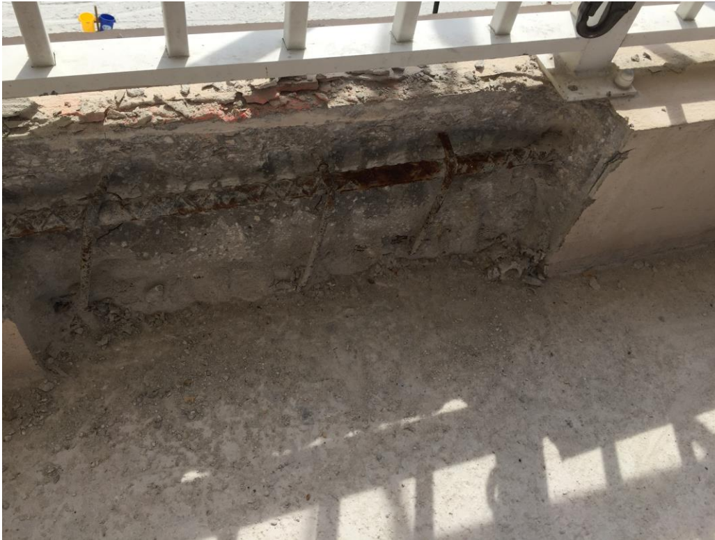
Picture 3: Typical curb excavation
